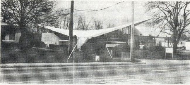
BANK ONE, 7112 East Main Street. The most unusual building in the city, the roof shape is a hyperbolic paraboloid. It was built in 1960.
