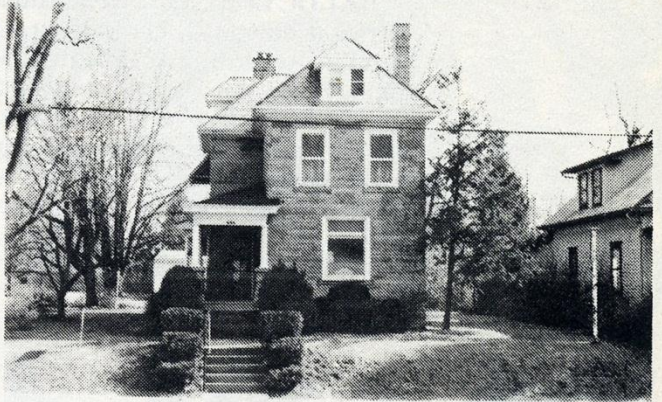
HOUSES, 7645 East Main Street and 1292 Lancaster Avenue. These are the only houses in town built entirely of stone from William Forrester's quarry on Waggoner Road. The cut blue freestone was popularly used in the county for lintels and doorsteps. The quarry was opened by Henry Besse, who took possession of his land in 1828; was later run by George Graham and then by Forrester.
