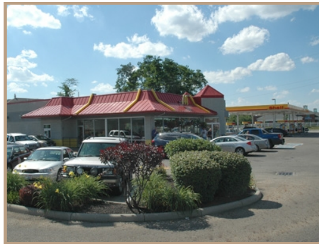
McDonalds/Shell now sits on this same stretch of St. Rt. #256, just north of the I-70 Interchange.
