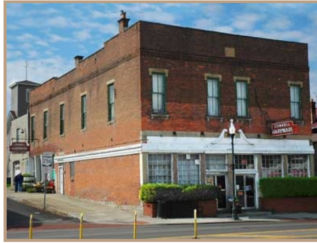
Here is Connell Hardware in this 2009 photo. The main entrance is now on the Lancaster Avenue side of the building.
